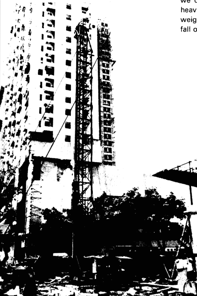
Pile driving with a 'drop hammer'
